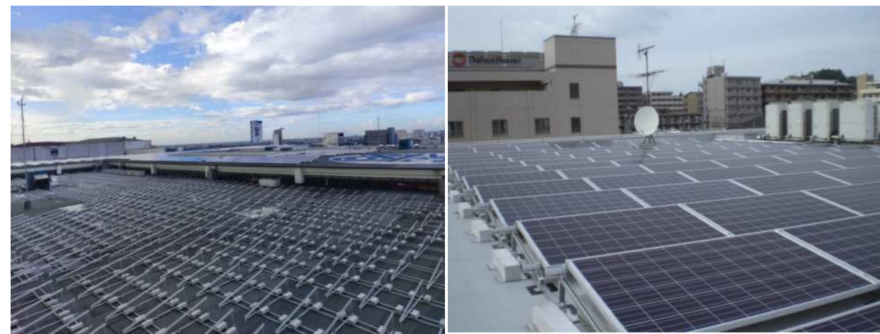
Ballast Bracket System
