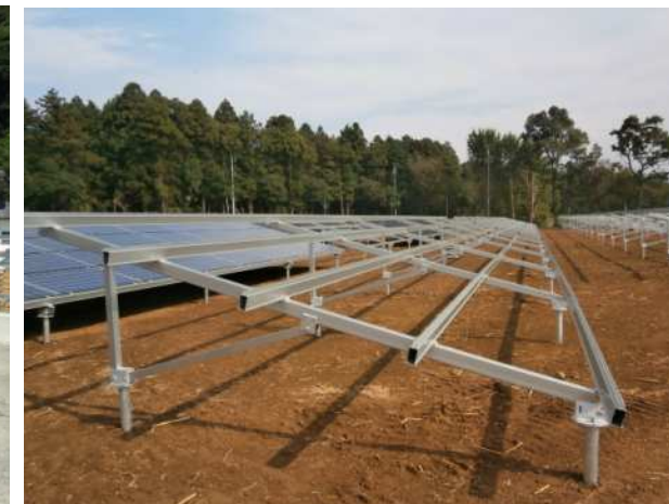
Ground Screw Foundation
