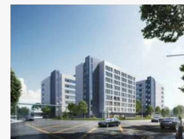
Production Center II 45000 m 2
